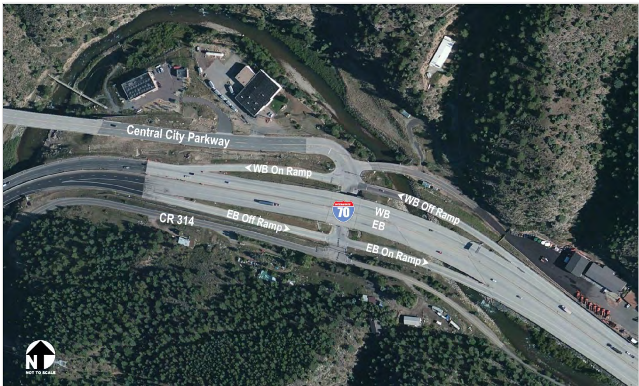
Exhibit 9. Exit 243 (Hidden Valley/Central City) Interchange
